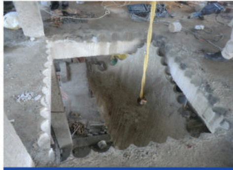
CONCRETE SLAB CUTTING
